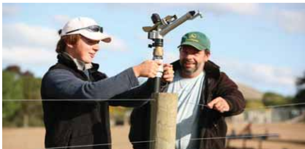
Harry and Haydn working on the new irrigation system.
